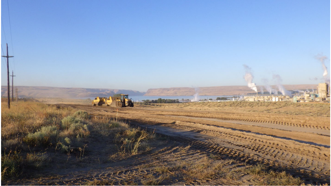
Figure 1. Scraping and widening of the existing E. Attalia Road, view to the southwest.
