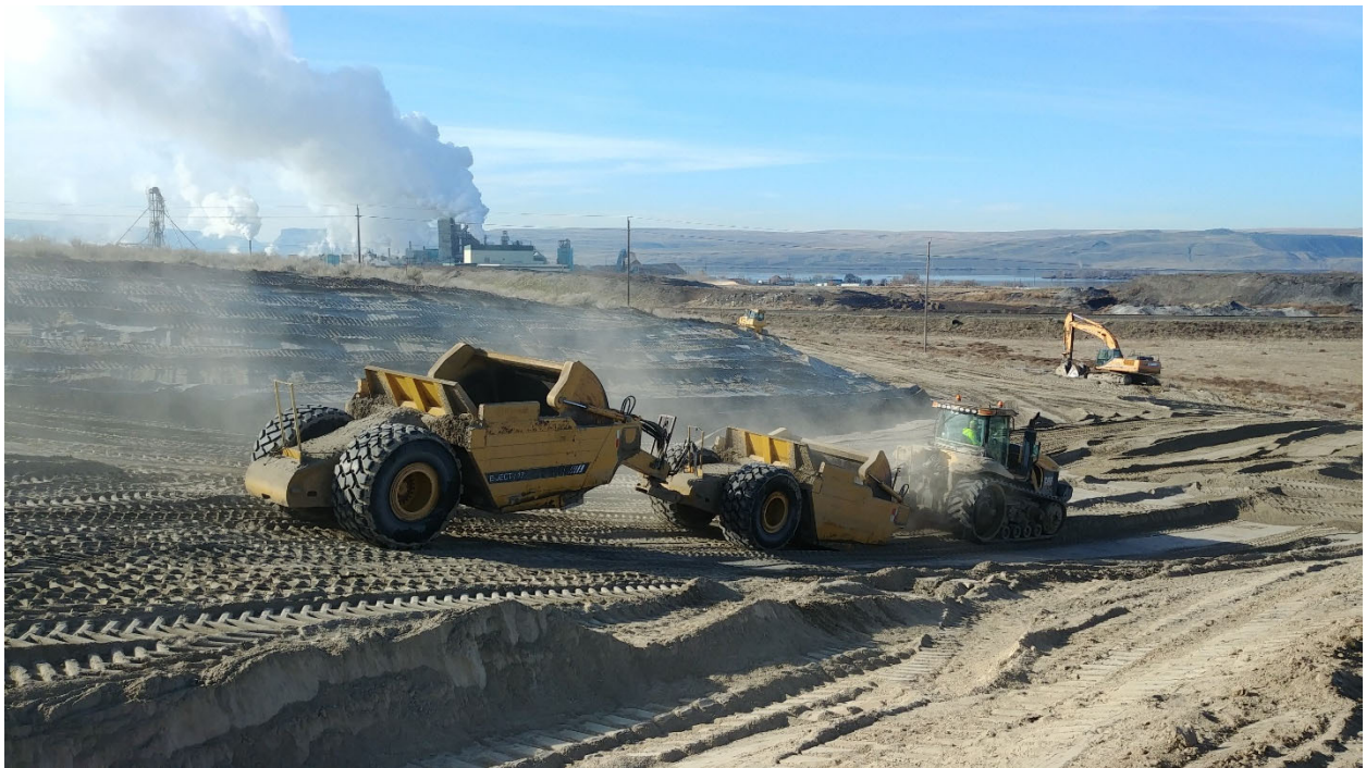
Figure 2. Deep scraper cuts that connect the improved E. Attalia Road and Sundance Road, view to the southwest.
