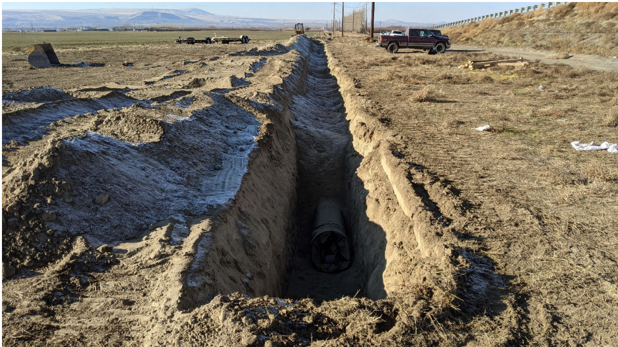
Figure 20. Trenching and installation of distribution main along Dodd Road, facing west.
