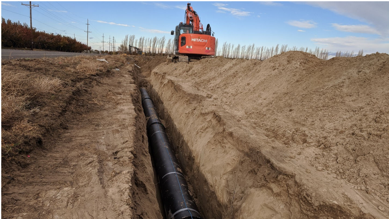
Figure 18. Trenching and installation of 18-inch (in) distribution main along Railex Road, facing north.
