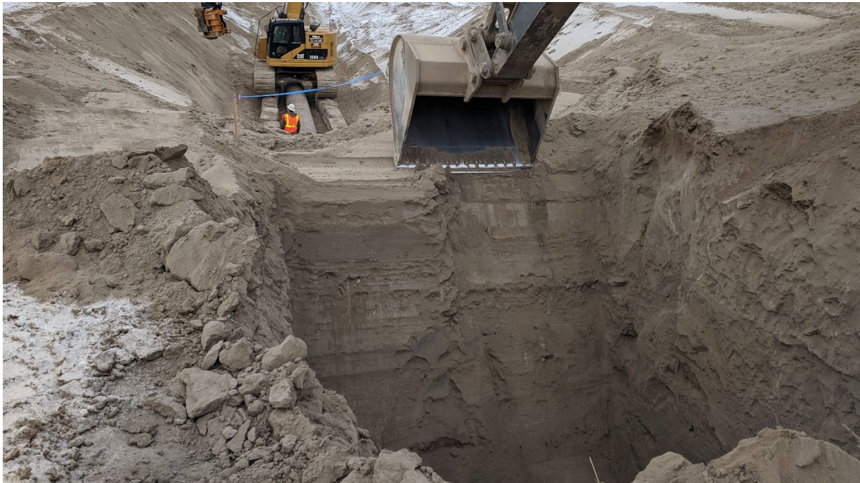
Figure 9. Beginning excavation of the 17-foot trench that connects the A-Line and B-Line, view to the south.
