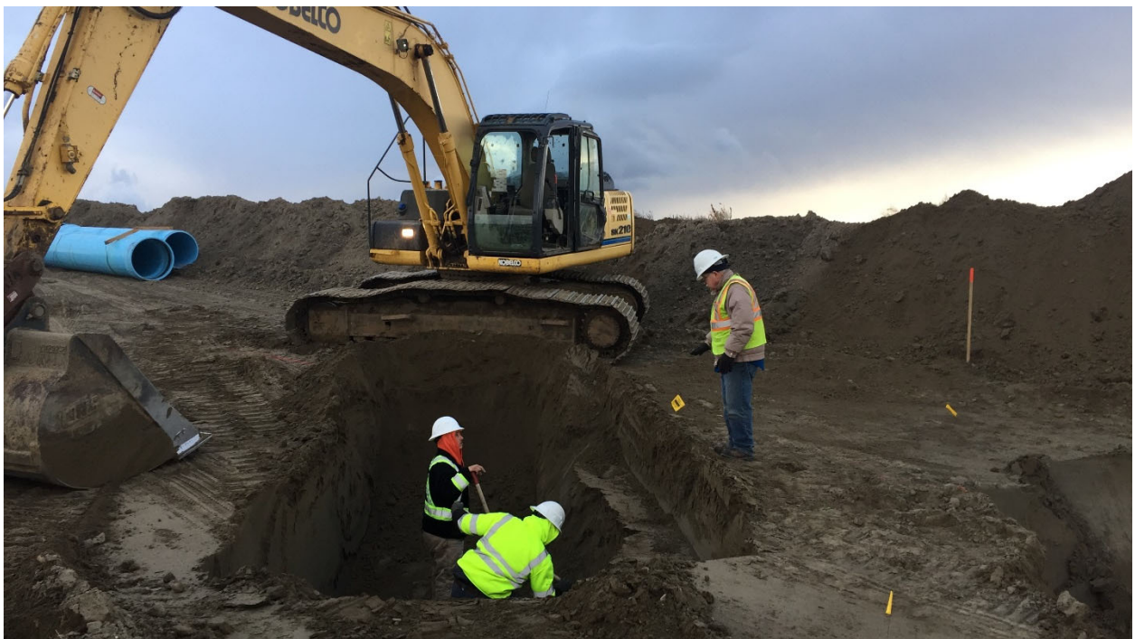
Figure 8. Beginning of potholing for the two Marathon Pipe Line LLC liquid petroleum lines, view to the southeast.
