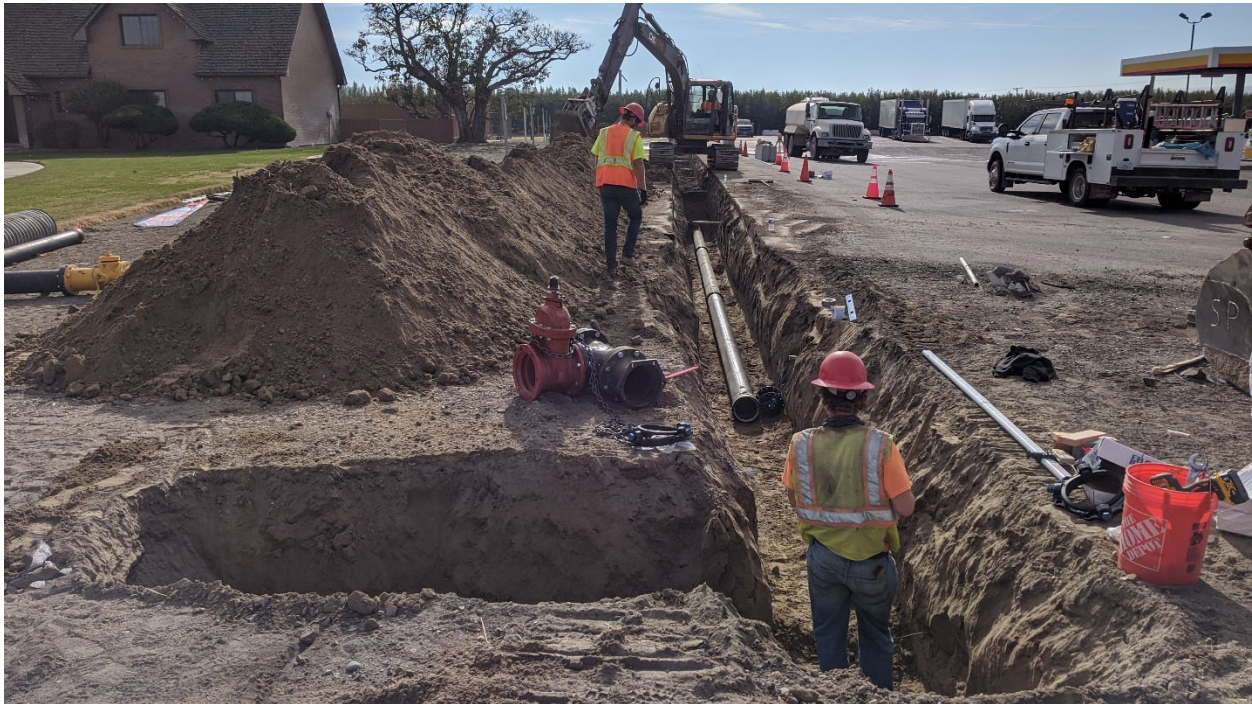
Figure 19. Trenching and installation of 8-in distribution main in Shell parking lot, facing south.
