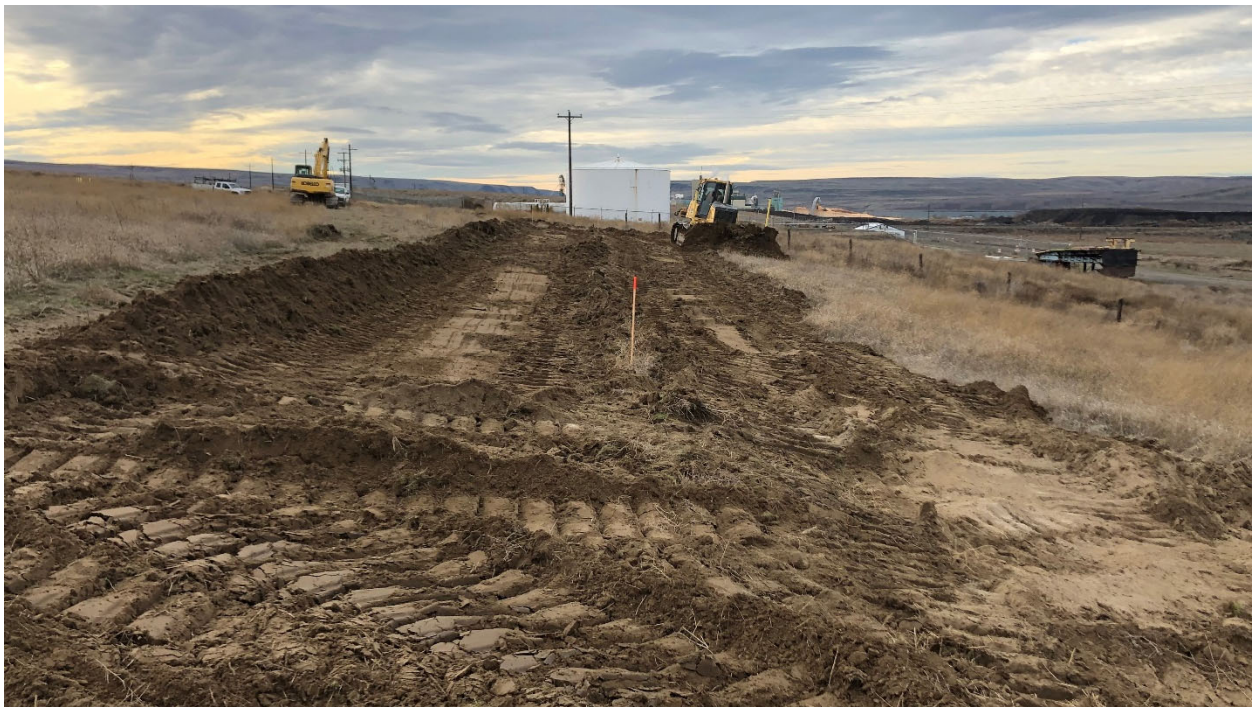
Figure 6. Grubbing operations for the B-Line, facing southwest.
