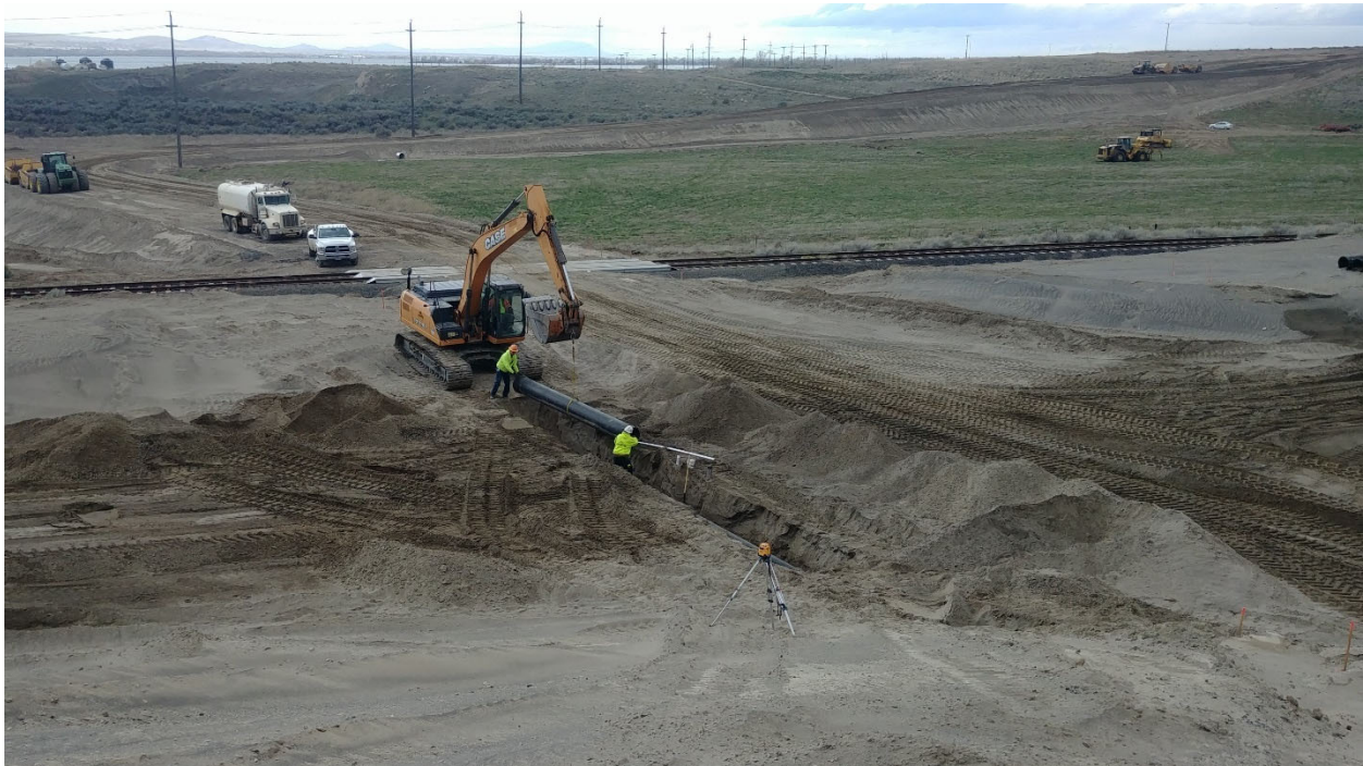
Figure 5. Overview of high density polyethylene pipe installation under Sundance Road, view to the northwest.
