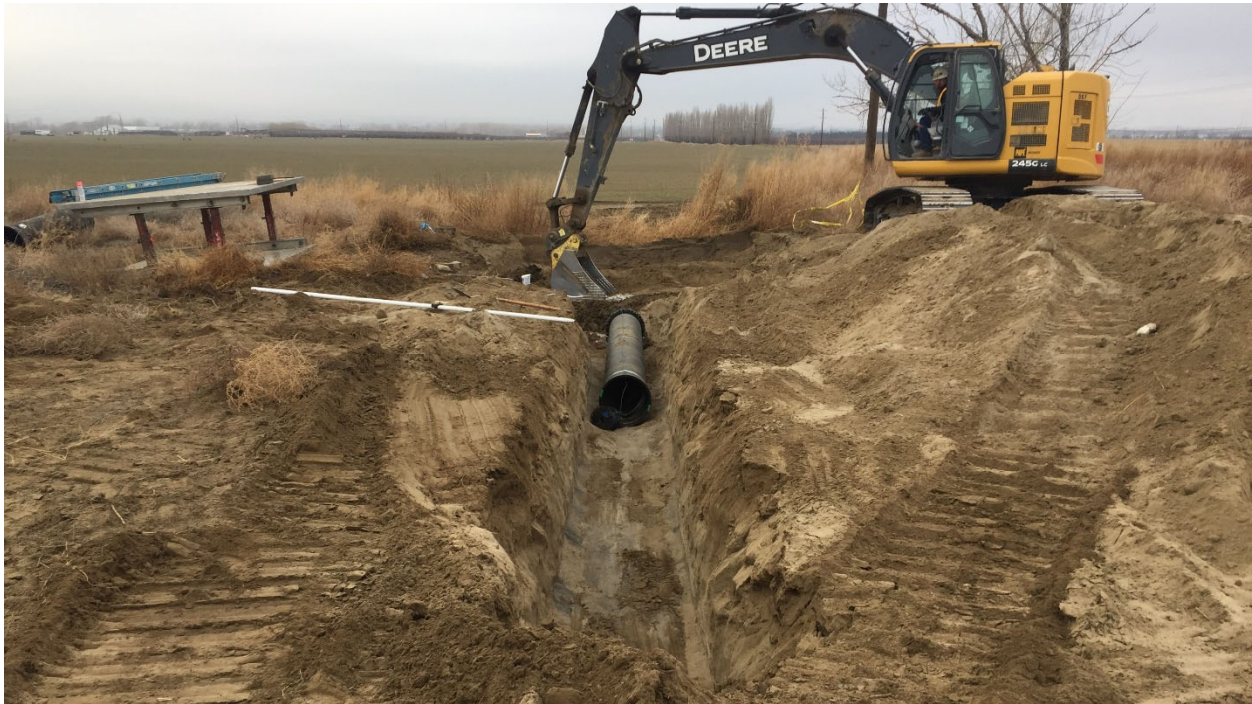
Figure 21. Trenching and installation of distribution main between Two Rivers East Lateral and Tyson Fresh Meats, facing west.
