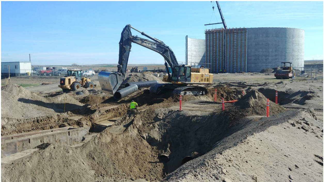
Figure 14. A-Line to swale installation near the concrete reservoir, view to the northeast.
